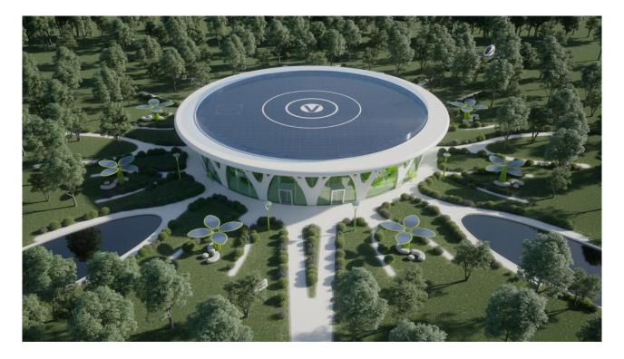
Large structural trees over 6 m high, made by WASP in eco-cement 3D printing, will support with their branches an extensive photovoltaic roof capable of generating 200 kWp energy and collecting and accumulating rainwater, which can then be used for irrigation of the park. In addition, thanks to the collaboration with eVertiSKY the roof will become a small vertiport, equipped with a telescopic lift and landing platform for electric passenger drones, useful for observing the forest from above.
